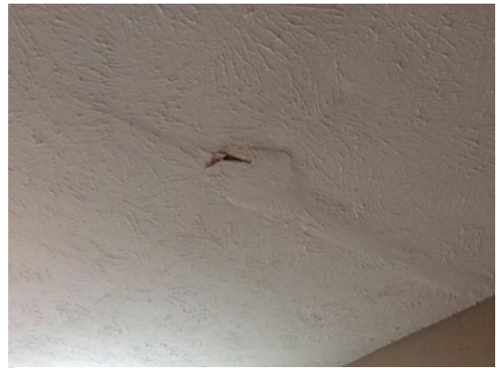
Ceiling (Hole and discoloration in ceiling)
