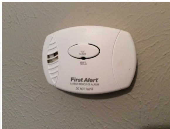
Carbon Monoxide Detector
