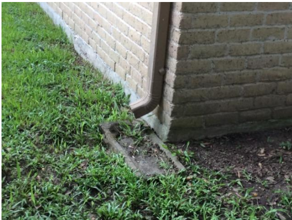
Downspout/ Splash Blocks
