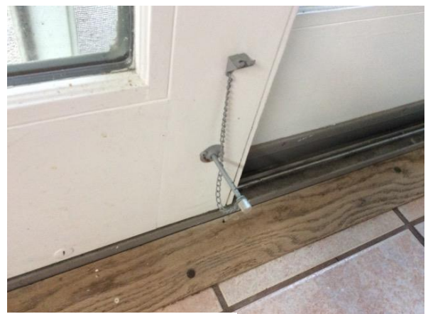
Sliding Door/ Pin Lock
