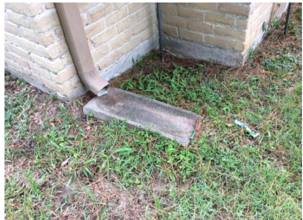
Downspout/ Splash Blocks
